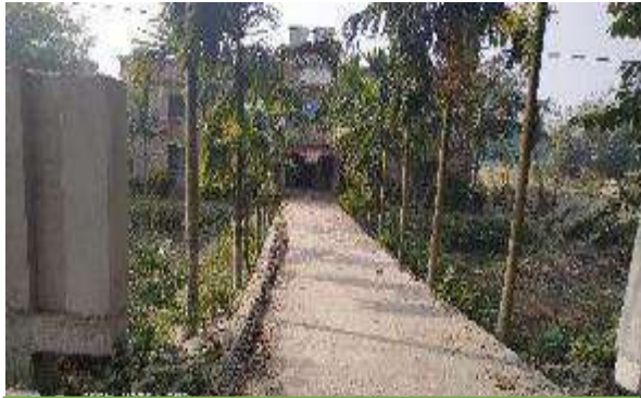
Approach road and boundary wall at Arua UH&FWC, Manikganj
